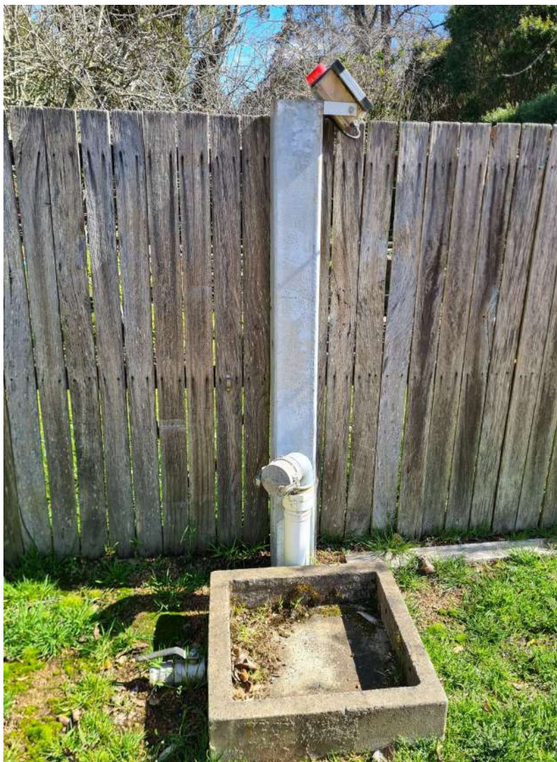
FIGURE 4 EXAMPLE OF SPILLAGE PIT UNDERNEATH A PUMPOUT STANDPIPE
